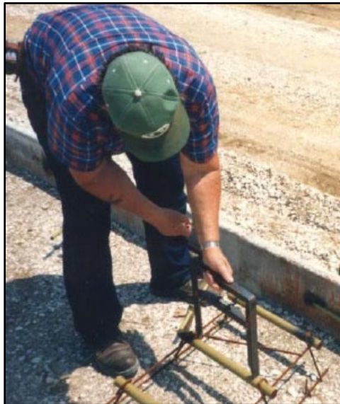
Figure 8.10.1. Dowel Bar Checker Device
